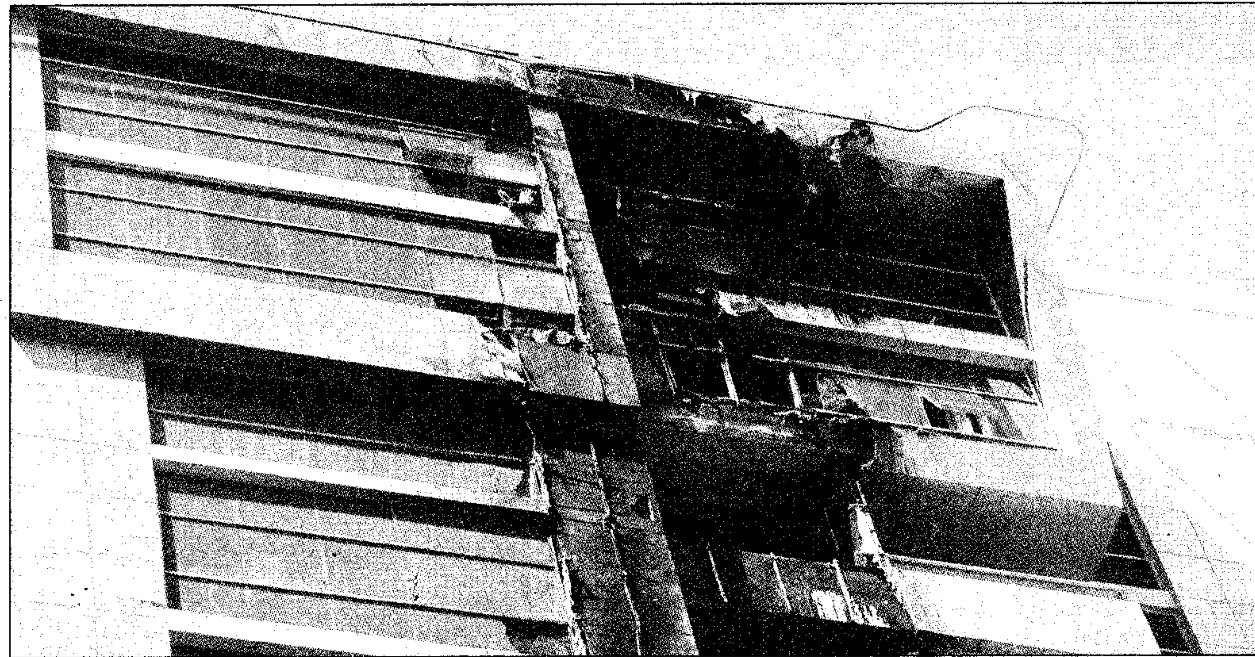
GUTTED: The burnt out apartments that spread from the fourth to the ninth floor of the Tecom tower
